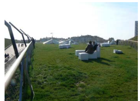
The walkable part of the green roof is equipped with comfortable seats for relaxing.
