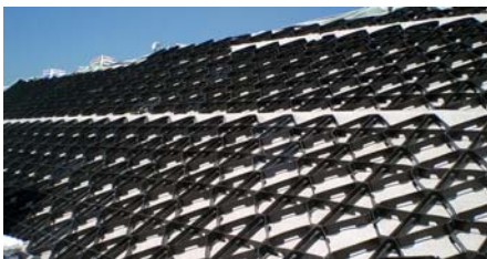
Installation of the Georaster® elements on the steep roof.
