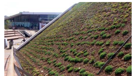
The steep roof with the different species of Sedum.
