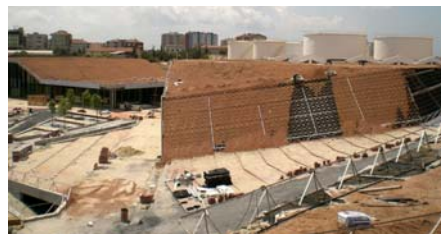
The Georaster® infilled with System Substrate.
