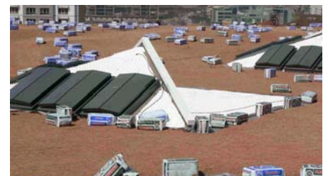
The thickness of the substrate layer at the Meydan Centre is 100 mm.
