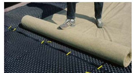
Floradrain® FD 25-E and Filter Sheet SF are installed.
