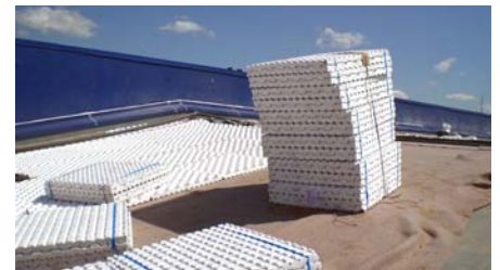
Installation of the drainage elements Floraset® FS 75.
